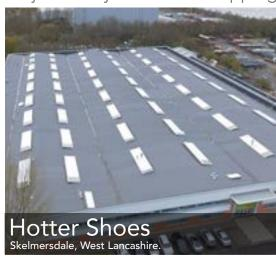
The roof on the Hotter Shoes' head office and manufacturing facility in West Lancashire had exceeded its serviceable life and was experiencing significant water ingress.
