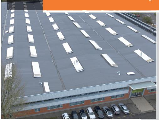
The waterproofing on Hotter Shoe's 12,500m<sup>2</sup> roof had exceeded its serviceable life and was experiencing significant water ingress, requiring urgent remedial work.
