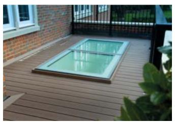
The rooflight is set into the structure to allow adjacent decking or paving slabs to be set level and sit flush with the top face of the rooflight unit ensuring a smooth surface. Care must be taken in wet or icy conditions. Etched glass can offer additional safety.
