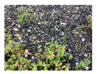
Make sure blankets are butted up tight and joints as neat as possible. Fill all gaps with substrate.
