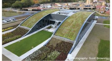
The roof slopes downward and fully integrates with the landscape; an aesthetically pleasing design, though not without its challenges. At some points, the curve of the roof reaches a pitch of over 30 degrees, meaning careful consideration had to be given to not only the type of waterproofing system and green roof finish, but also to safe installation.
