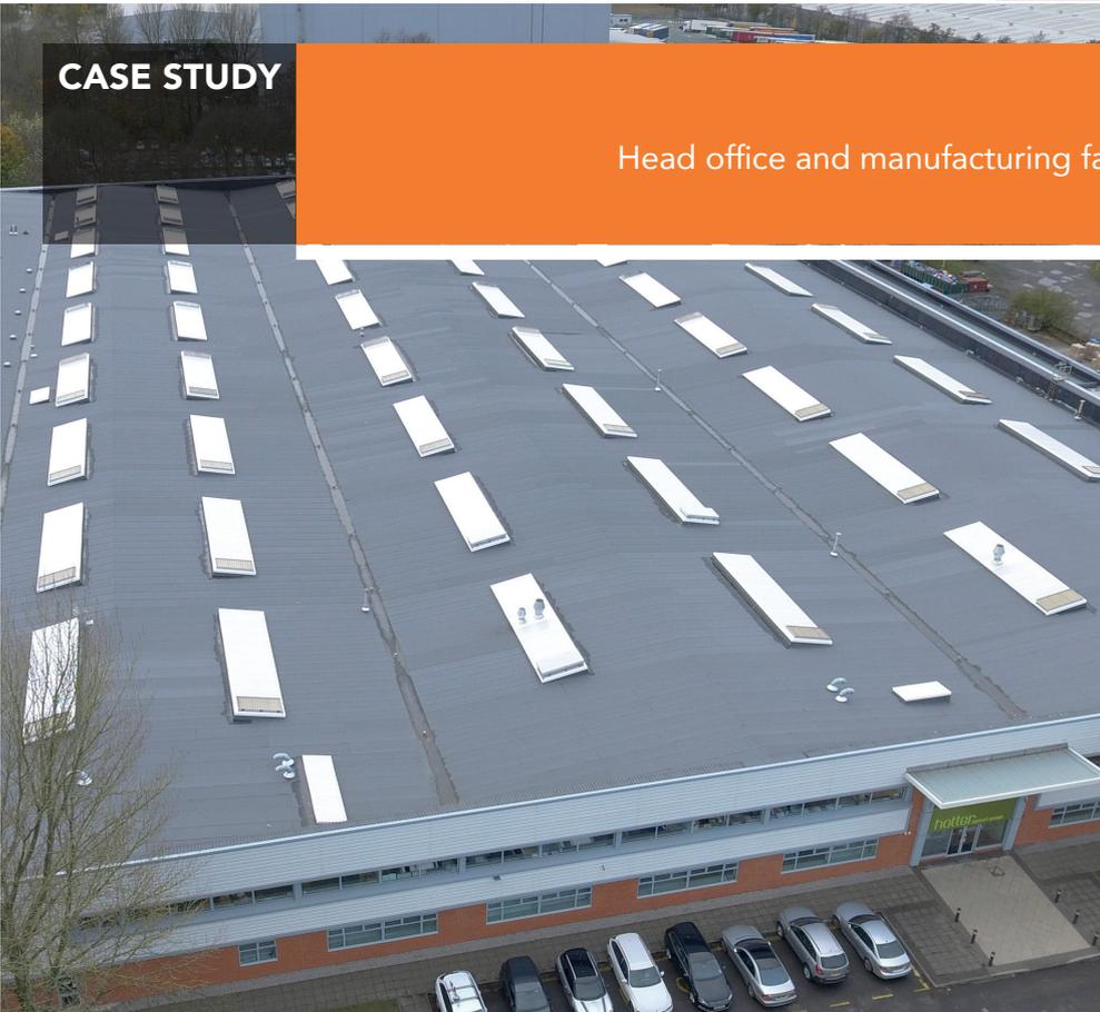
The waterproofing on Hotter Shoe's 12,500m<sup>2</sup> roof had exceeded its serviceable life and was experiencing significant water ingress, requiring urgent remedial work.
