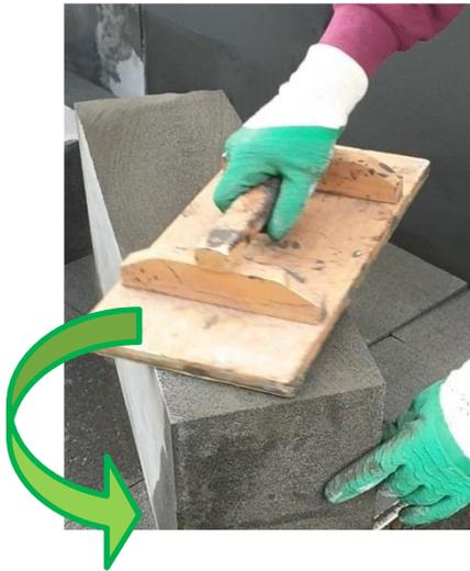
Use a sanding block to shape the underside of the insulation, to ensure a firm and stable contact with the substrate or an abutment.
