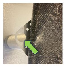
When fixing through existing outlets, the long outlet spigot should extend beyond the spigot of the existing unit to from a seal with the downpipe beyond and should then be cut to the length required.
