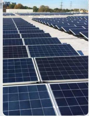
Tilley Roofing overlaid the original single ply waterproofing with over  $12,000m^2$  of Bauder's lightweight, robust PVC single ply waterproofing system Thermofol. The solar modules, which weigh less than  $12Kg/m^2$ , were then fitted using a unique penetration-free method by renewable energy specialists Dulas.
