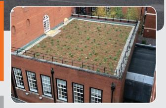
The building consists of 12 different roof areas totaling over 1,200m<sup>2</sup>. All of the original waterproofing on the main roof areas was removed before being replaced with Bauder's reinforced bitumen system, which included PIR insulation. On the building's lower roof, located in the central courtyard area, 200m<sup>2</sup> of Bauder's premium
