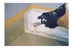
For internal corners bring the fleece 50mm around the corner and cut at the base of the fold into the corner. Overlap the cut section, making sure that there are no dry fleece overlaps.
