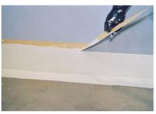
**TIP:** For high upstands and upstands with height changes use wider sections of fleece applied in vertical strips to ease application.
