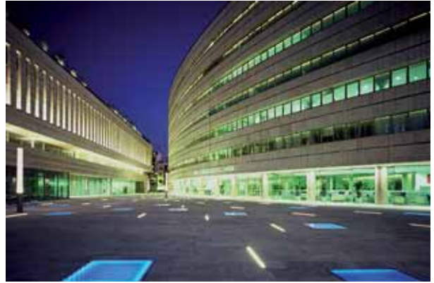
DPH Pedestals supporting large format marble slabs
