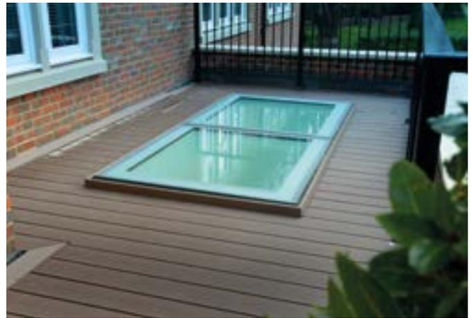
The rooflight is set into the structure to allow adjacent decking or paving slabs to be set level and sit flush with the top face of the rooflight unit ensuring a smooth surface. Care must be taken in wet or icy conditions. Etched glass can offer additional safety.
