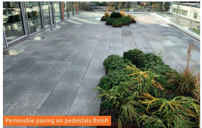
Permeable paving on pedestals finish
